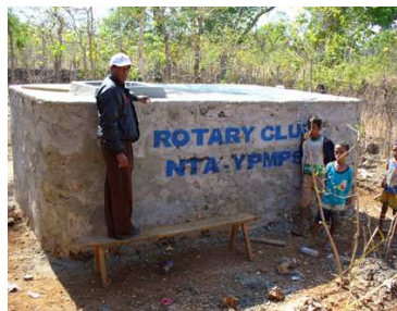
Concrete 15,000 litre off-roof water tank
